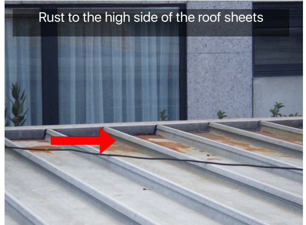
The roof is badly rusted
