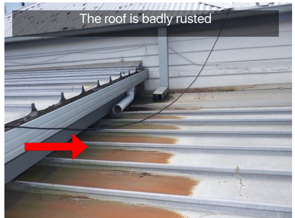
The gutters to the shed need to be replaced
